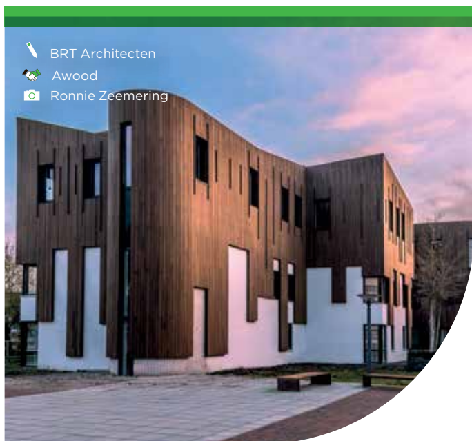
Notiz Hotel NHL Stenden - Bamboo X-treme® Cladding installed to reflect the “dressing” of a chocolate cake - (1200 m²) Leeuwarden, The Netherlands
